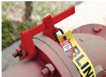
Blind Flange Lockout
