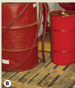
Violation: Not compliant spill pallet
