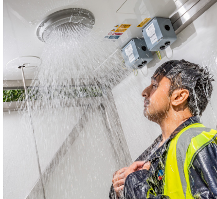
Compliant spray pattern ensures a thorough decontamination of the casualty
