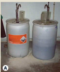
Violation: Hazardous liquids, no spill protection
